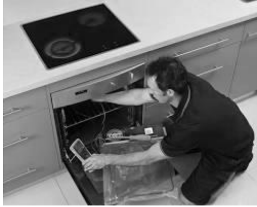
Installed electrical cooker
